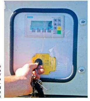
The driver places the RFID tag in front of the read/ write head, which reads all the relevant data and forwards it to the control systems
